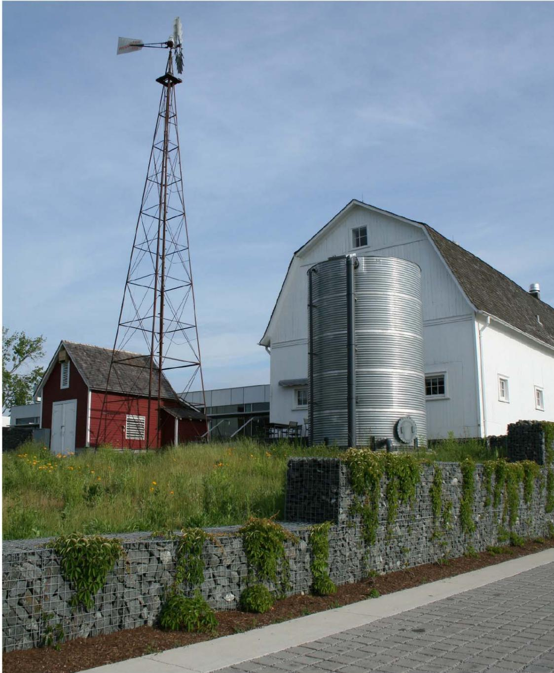
The entire site landscape thrives without the use of potable water. Rainwater is harvested, treated, and stored in a 15,000 gallon cistern to provide make-up water for the wetland, and supplemental irrigation water for the green roof system. A dining patio is perched next to the barn capitalizing on views down into the landscape.
