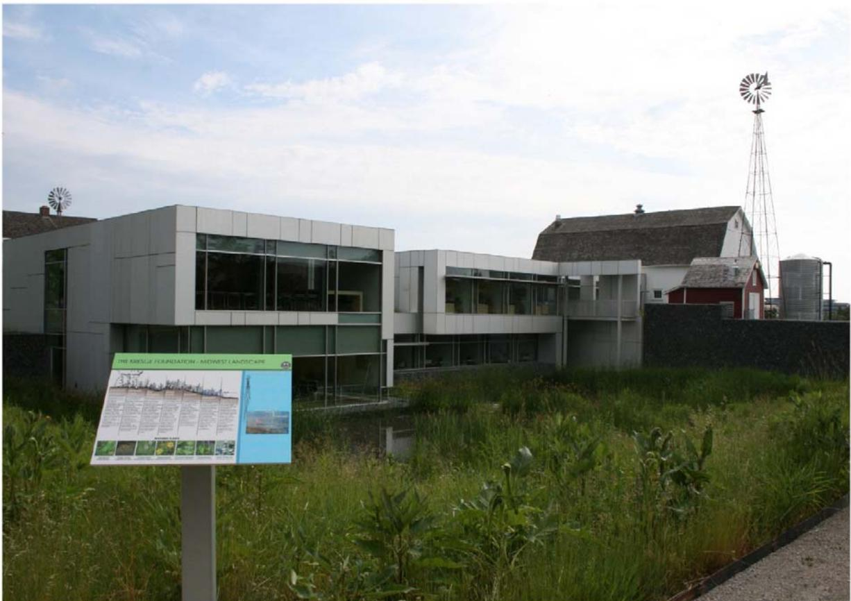
Water was a primary design consideration for the project. The created wetland, green roofs, porous pavement, bioswales, and rainwater harvesting and re-use are the primary components of the integrated rainwater system. Kresge added interpretive signs throughout the landscape to communicate these design principles.
